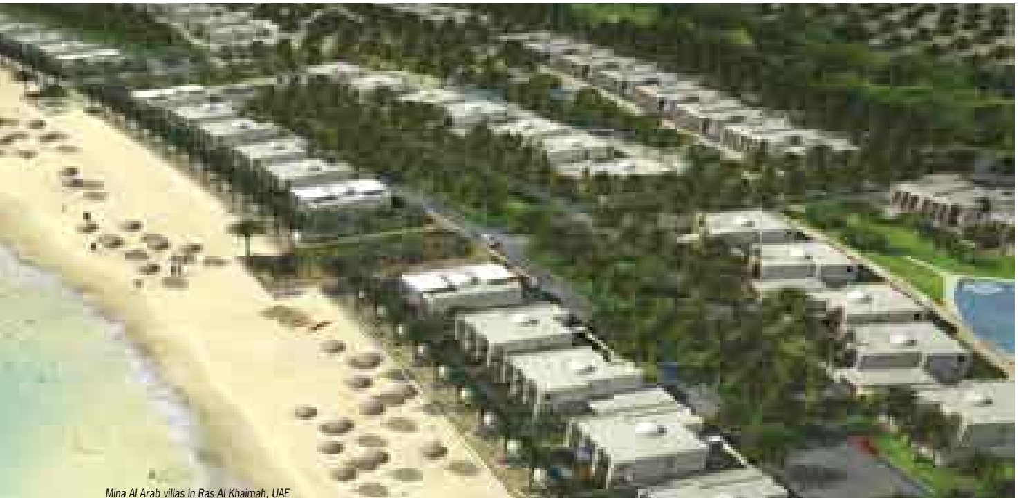
Mina Al Arab villas in Ras Al Khaimah, UAE
