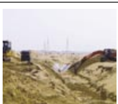
SNASCO, the master developer of the Sharjah Investment Centre, said that the third and final phase of the project is underway.
